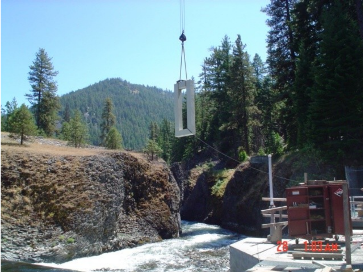
Figure 1. Castile Falls Fishway PIT tag system under construction.
